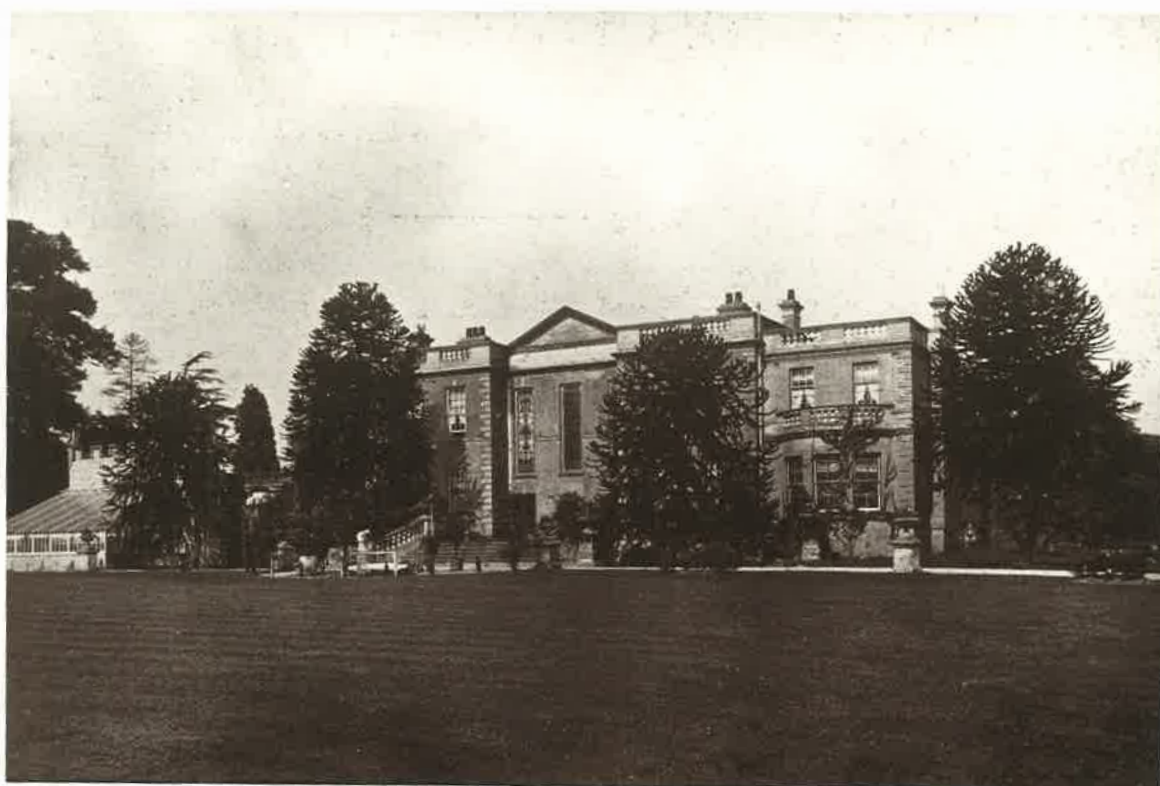
SOUTH VIEW OF HALL.
