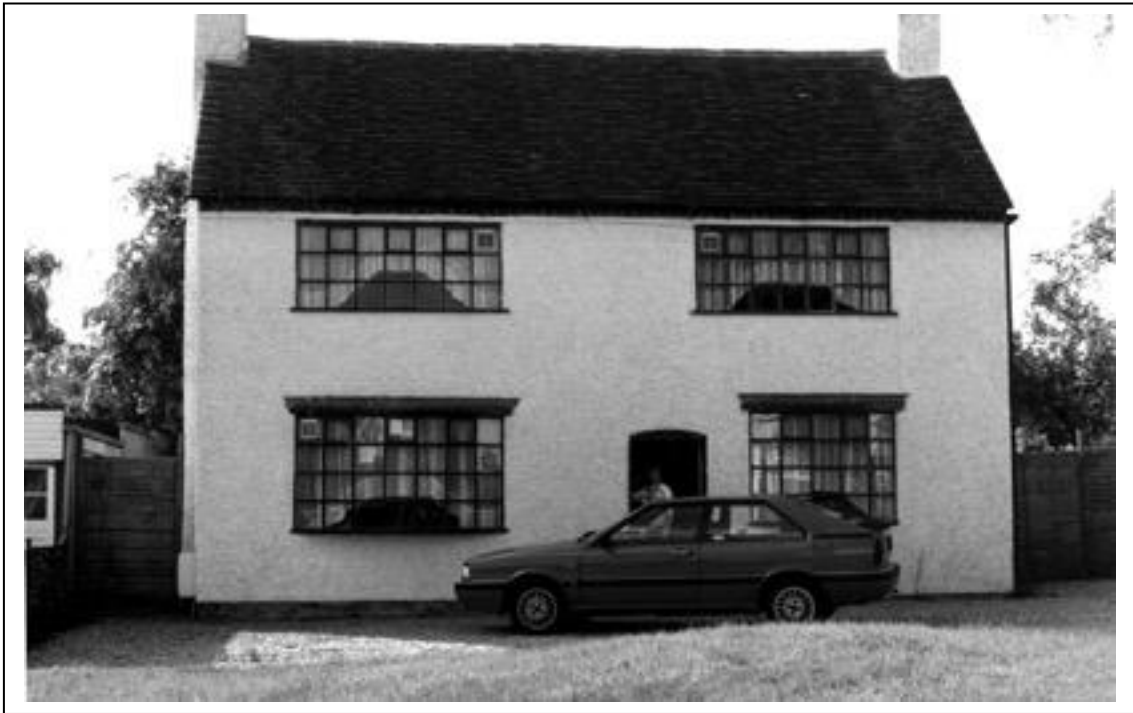
Photograph 17 Fir Tree Cottage, Station Road in 1987.
