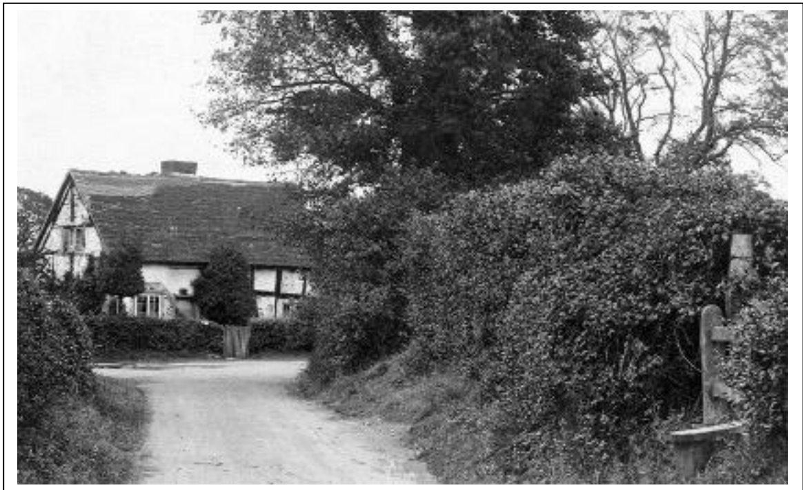
Photograph 71 Woodbine Cottage in Chelmsley Lane, looking down Alcott Lane.
