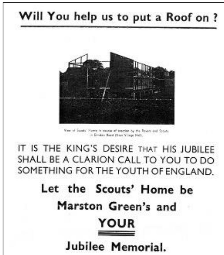
Figure 24 The leaflet asking for help to finish the building of the Scout Hut in 1935
