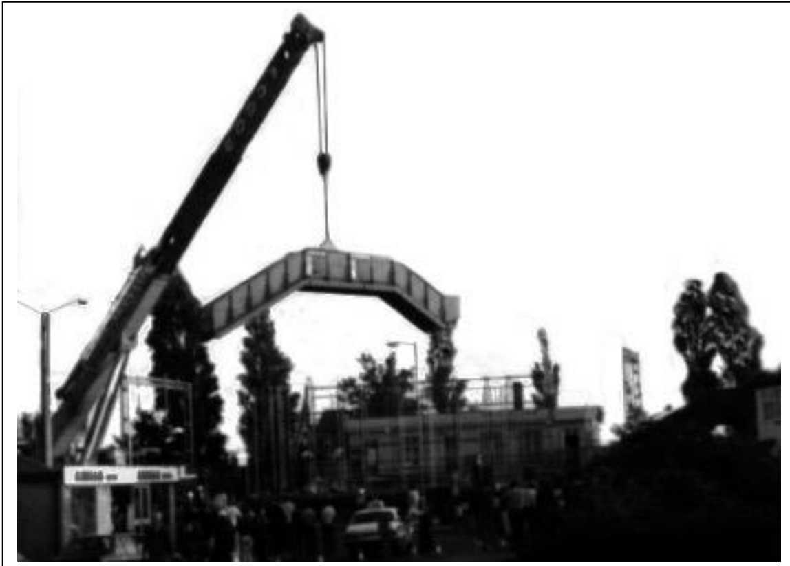
Photograph 120 The old bridge being removed from the station in 1984.
