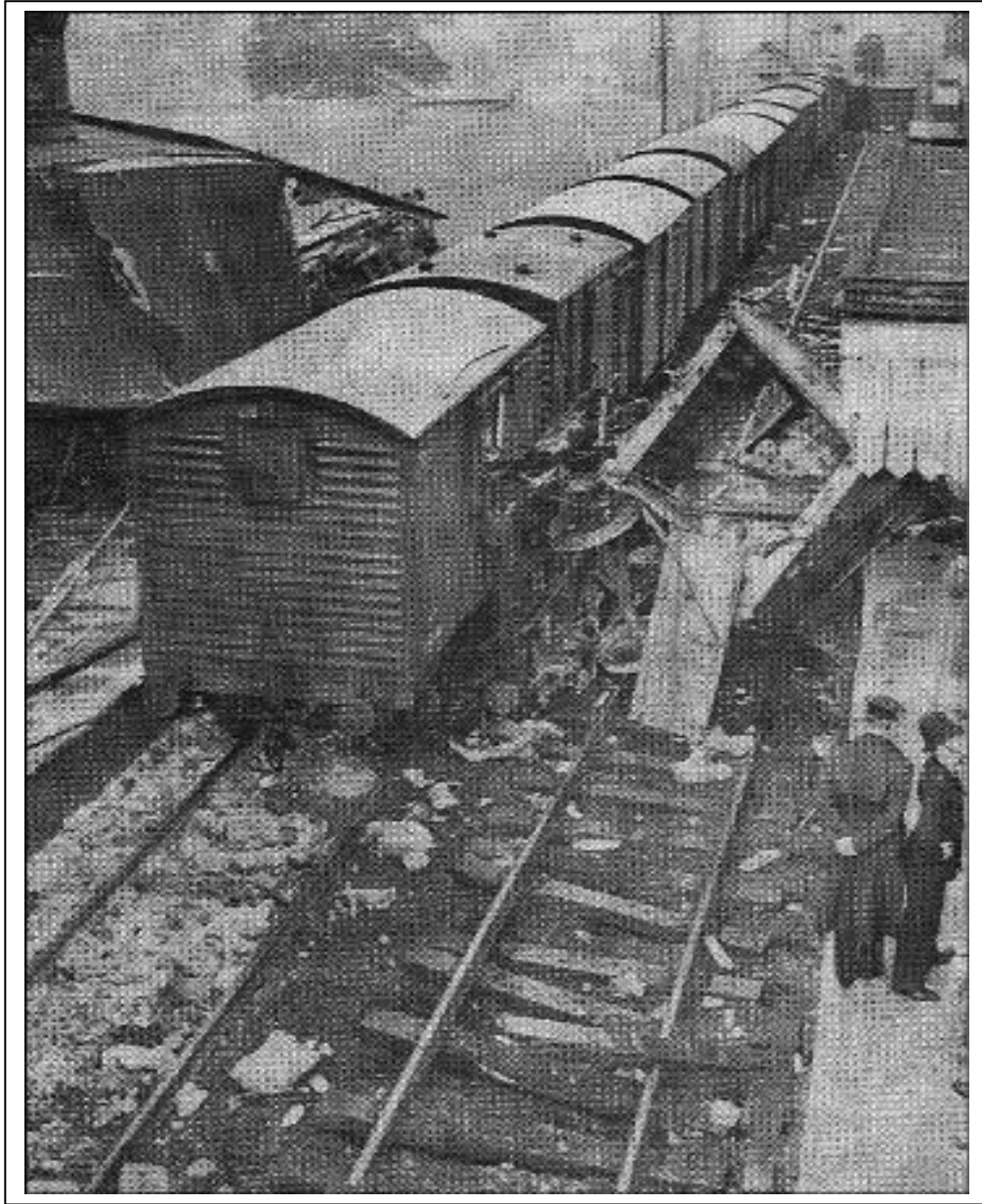
Photograph 85: Damaged track and platforms.
