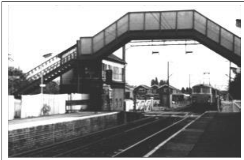
Photograph 81: The signal box and level crossing.
