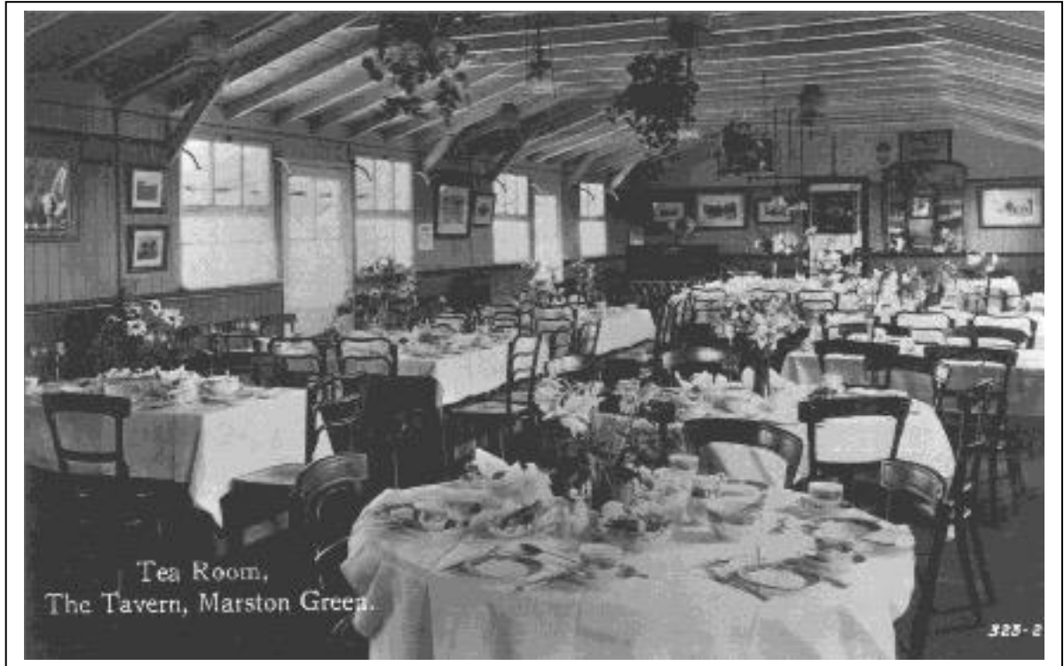
Photograph 28: The Tavern Tea Room.
