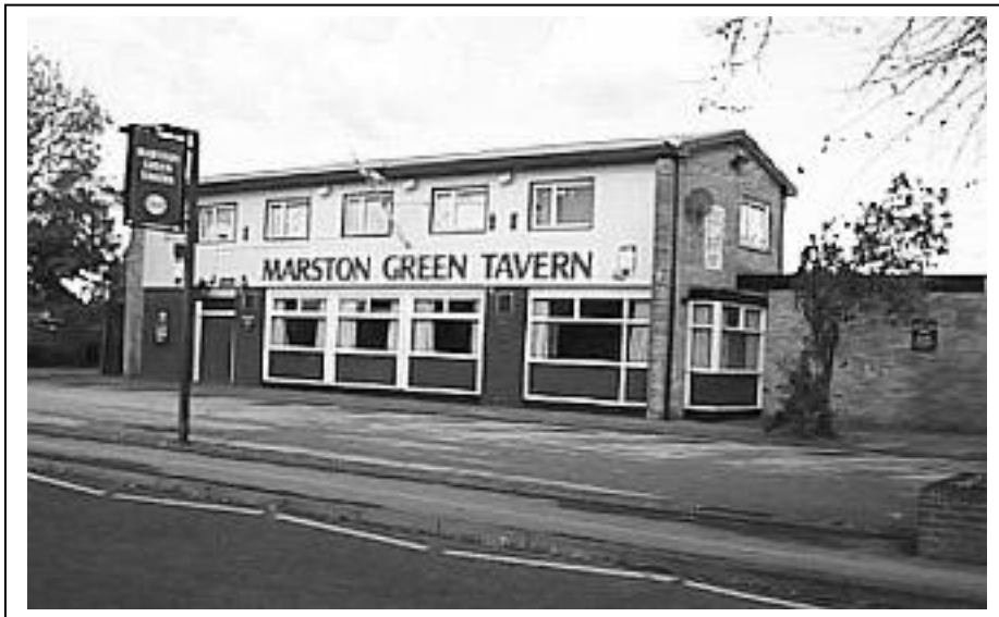
Photograph 23: The replacement modern Tavern. It was built in the early 1960's.
