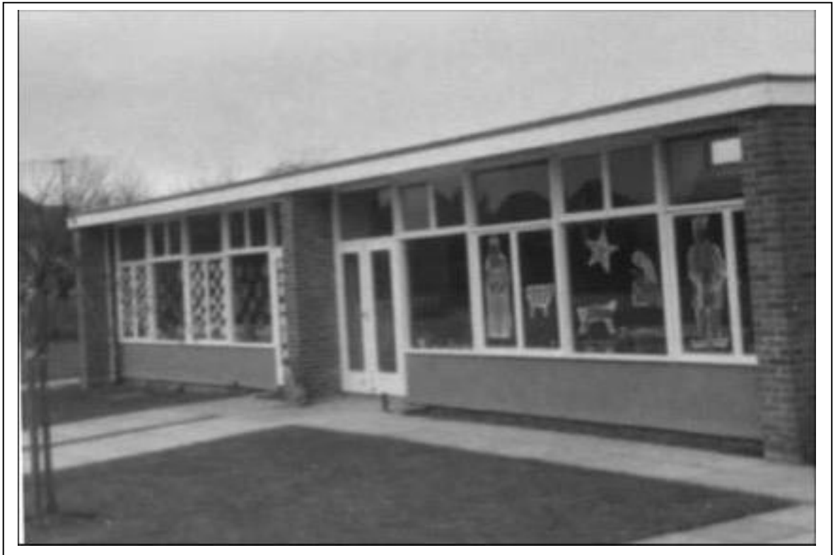
Photograph 53: The original Infant Classrooms - 1962
