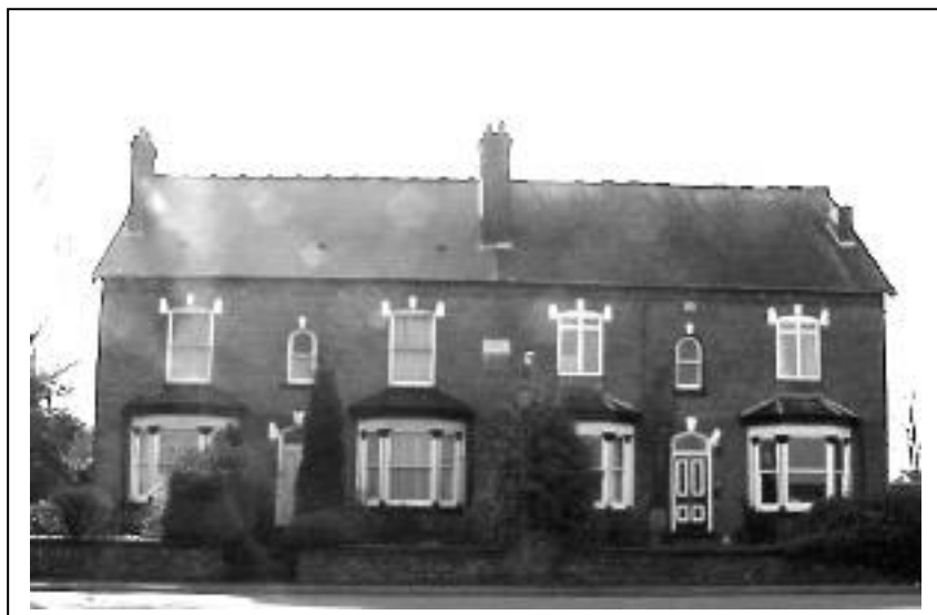
Photograph 90: Prospect Villas from the Church Car Park.
