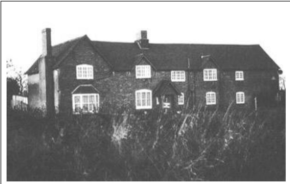
Photograph 130: Chapel House Farm.
