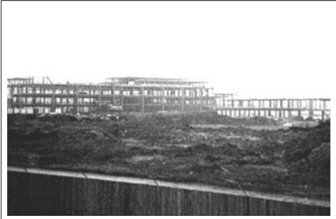
Photograph 78: Building work at Birmingham International Airport.
