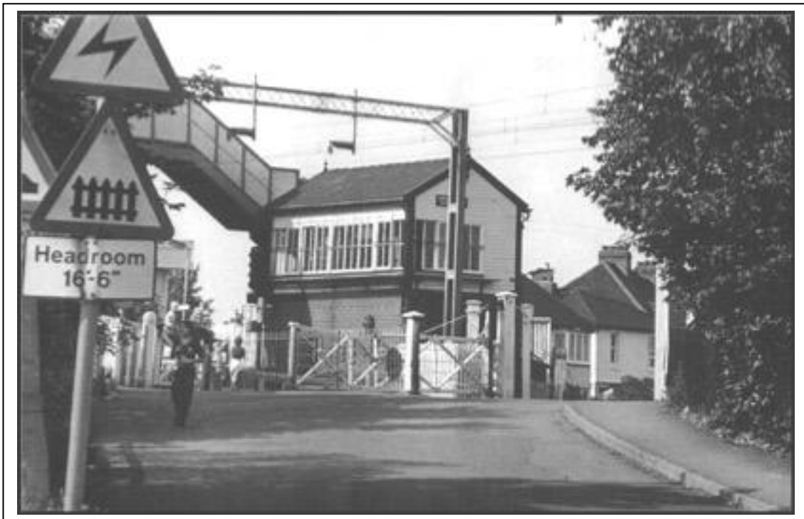
Photograph 12: The Level Crossing, seen from Elmdon Lane
