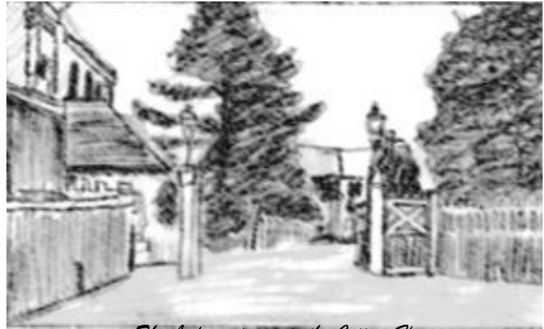
The Lodge entrance to the Cottage Homes.
