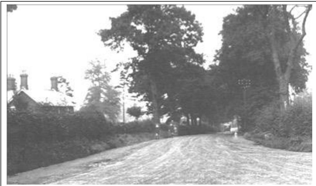
Photograph 95: Coleshill Road, Marston Green.
