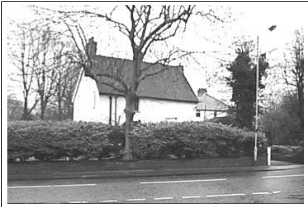
Photograph 125: The Old Police Station in Holly Lane.
