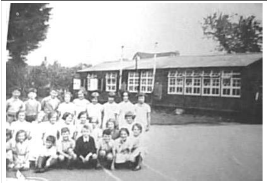
Photograph 47: The ex-army wooden classrooms.
