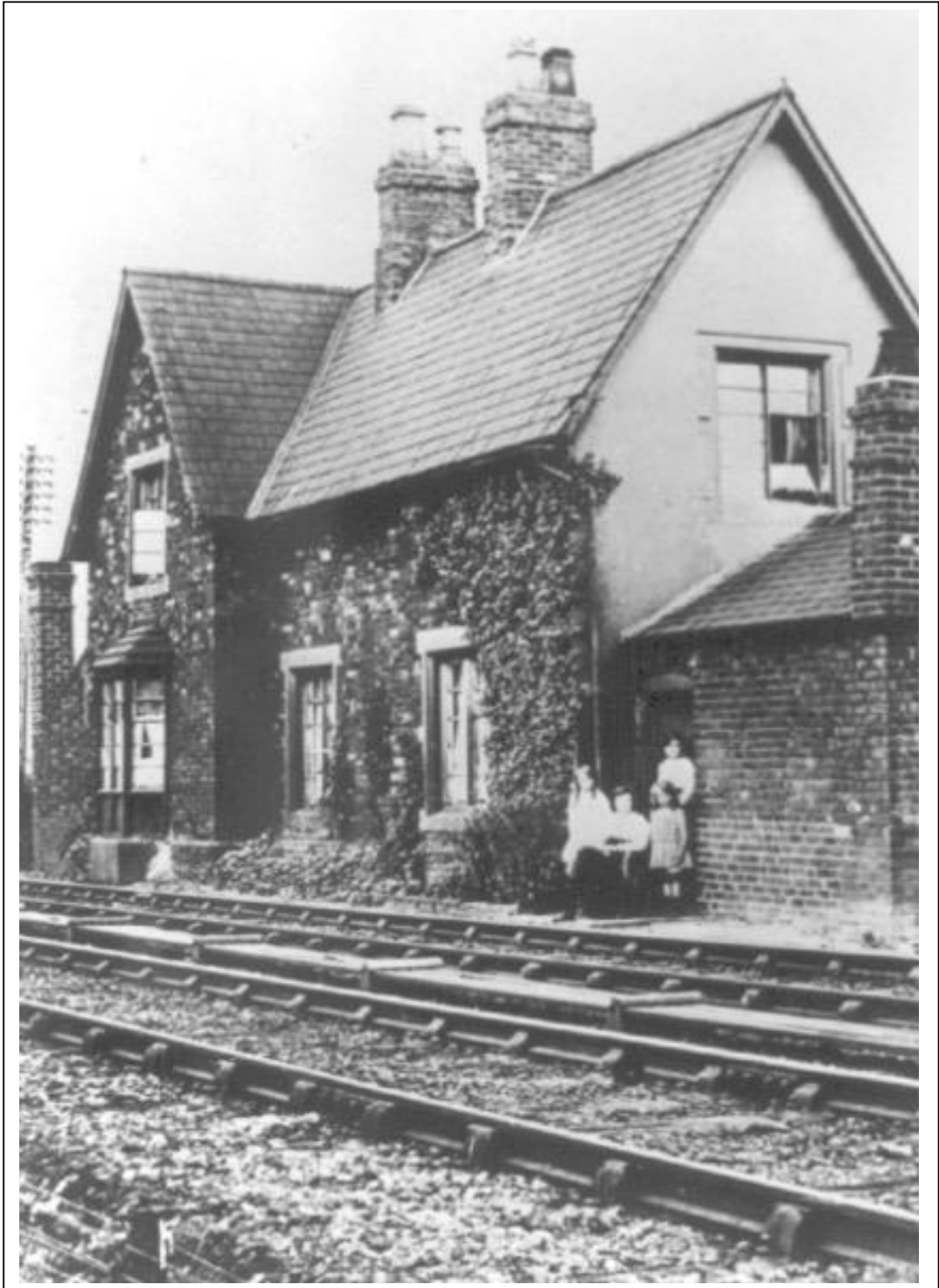
Photograph 110: The Station Master's House
