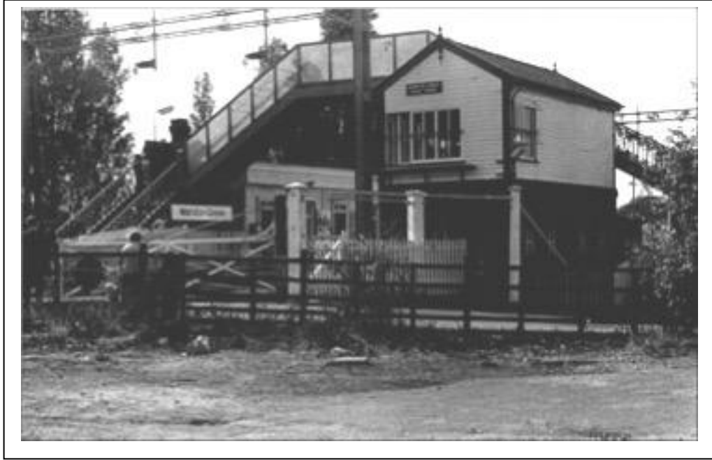
Photograph 80: The signal box at Marston Green Station. It is viewed from the Coal Yard (now the Station car park).
