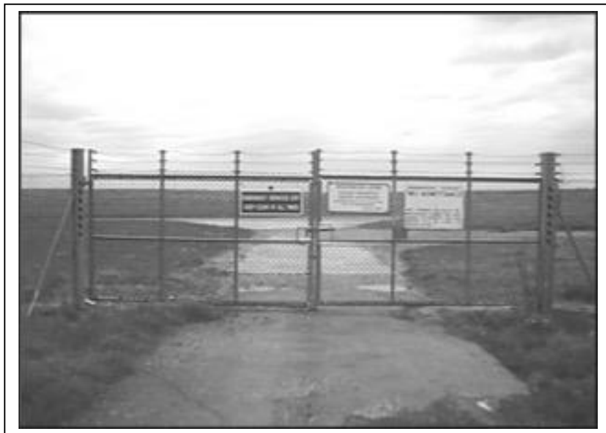
Photograph 14: Birmingham Airport Emergency Exit Gates The gates formed a no through road at the end of Elmdon Lane.
