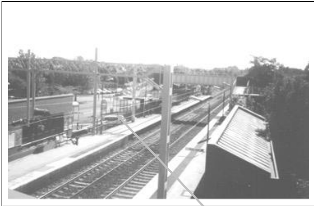
Photograph 82: Site of the level crossing and signal box. Both were removed in the 1970's.
