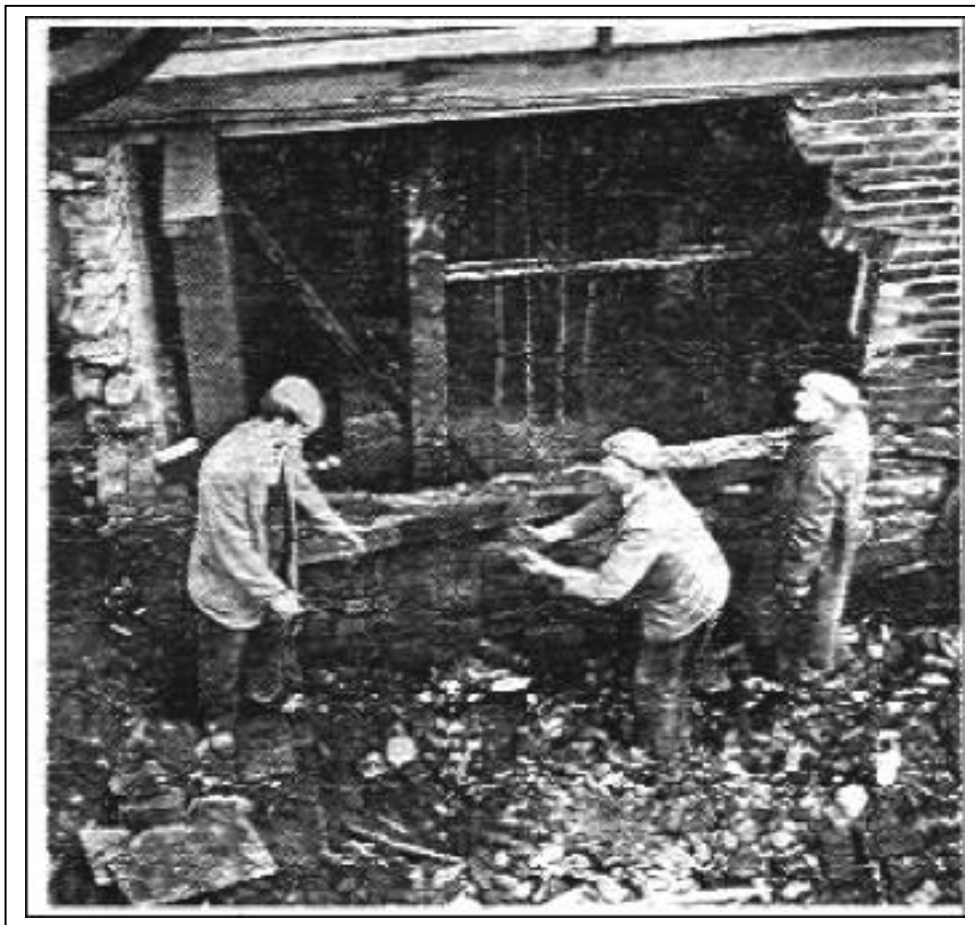
Article 12: Signal Box damage due to the Derailment.
