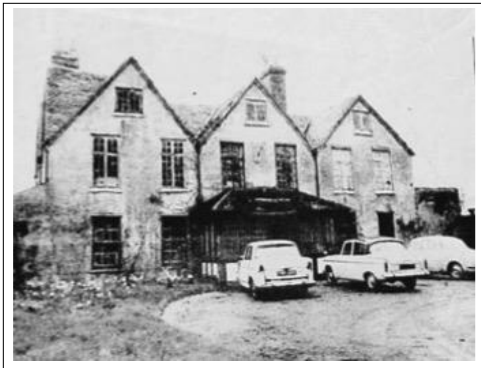
Article 11: Marston Hall prior to demolition.
