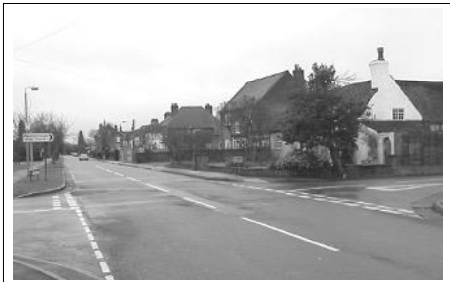
Photograph 112: Elmdon Road, late 1990's.
