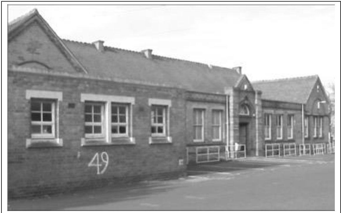
Photograph 71: The School at the Cottage Homes.
