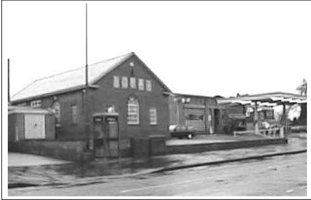
Photograph 134: The Telephone Exchange and Garage
